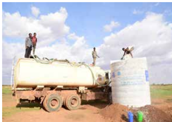
Fill the Amity sanitary storage tank with water under the supervision of the Local Water Board. (Figure 2)
