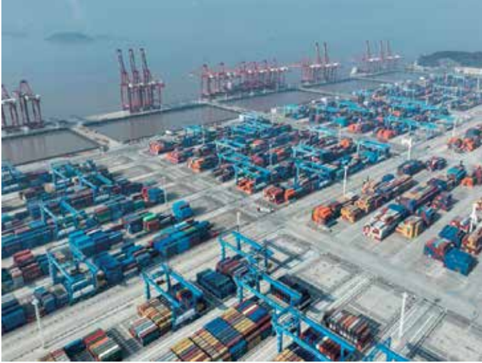
◀ An aerial drone photo shows a view of the container terminal of Zhoushan Port in Ningbo, east China's Zhejiang Province, on January 4, 2025 (XINHUA)
